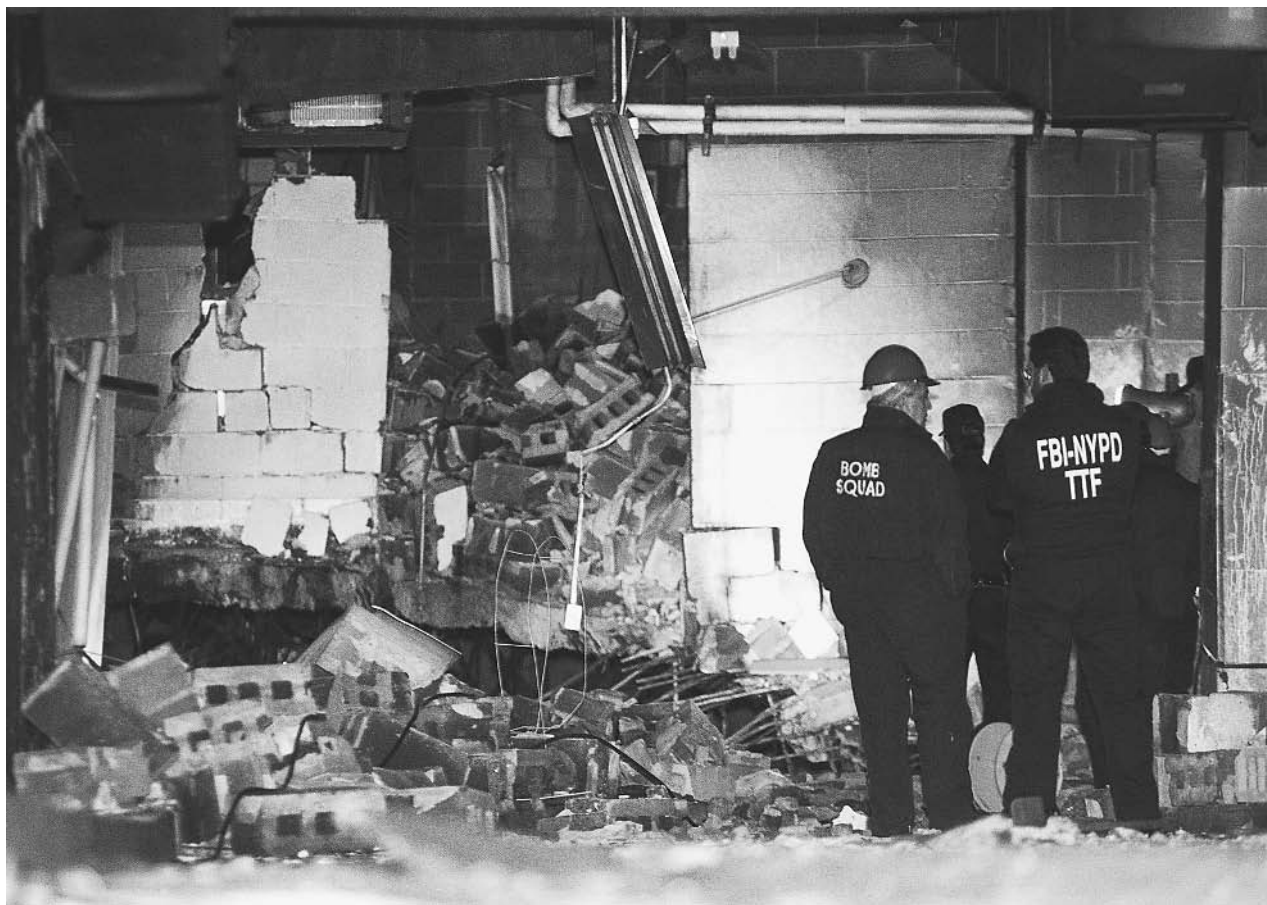
FBI agents view the damage caused by the 1993 terrorist bombing of the parking garage at the World Trade Center towers in New York. ©REUTERS NEWMEDIA INC./CORBIS.
